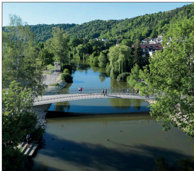
Fig. 4: Overview of the integral Duke's Bridge ( www.bergmeister.eu )
