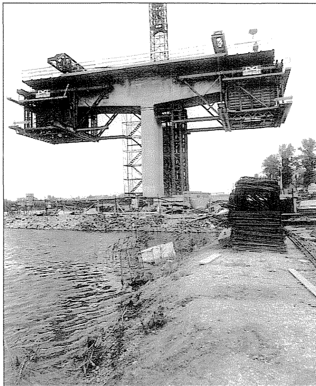
Fig. 2: Balanced cantilever method, M0 motorway, bridge over the Danube at Soroksár (1980).
