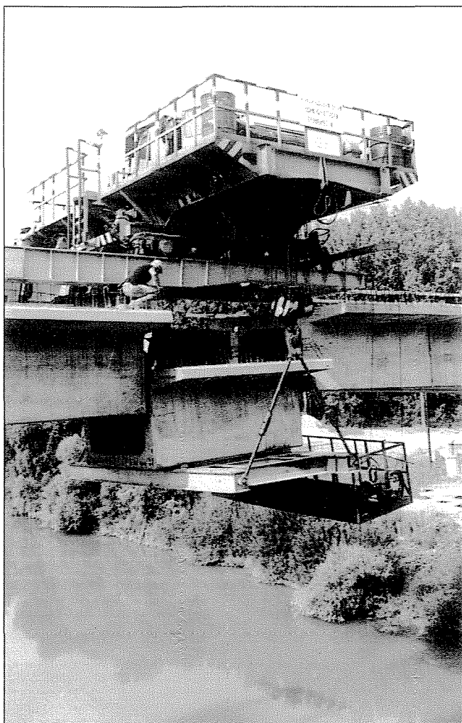
Fig. 1: The bridge over Hármas-Körös erected with the balanced cantilever method (made of pre-cast units), (1977).
