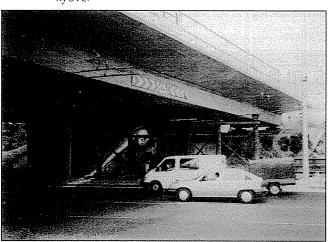
Photo 3 New pier under construction next to the existing flyover
