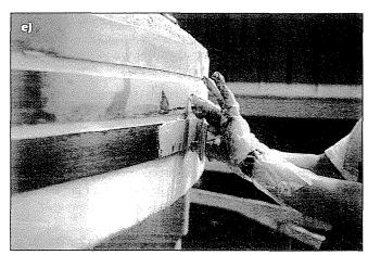
Fig. 6 Strengthening of a grain silo in Berettyóújfalu, Hungary, owing to the corrosion of circular prestressing tendons (Date: June 1997, Strengthening strips: Sika CarboDur S612-152 m. Designer: Dr. György L. Balázs. Exec: Isobau Rt.) a) Photo of the silo
