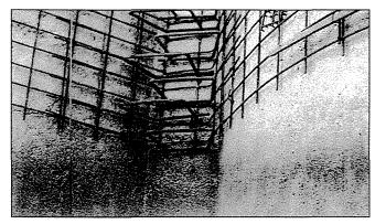
Photo 2 The anchorage and adjustment of wire mesh
