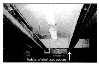
Fig. 4 Strengthening of a reinforced concrete beam owing to the elimination of an intermediate column in the Stollwerck Chocholate Fabric in Budapest (Date: July 1996. Strengthening strips: Sika CarboDur S512-44 m. Designers: Dr. György L. Balázs, Dr. István Hamza, Dr. György Visnovitz, Exec: ISOPLAN Ltd. a) Elevation b) Photo after strengthening
