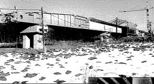
introduction. A number of upto-date, monolithic bridges with spare hollows were constructed on the section by-passing the city of Győr of the motorway M1. An important result of the technologic development was the introduction of the so-called incremental launching method. In the period from 1989 up to now yet 22 bridges were constructed by this method, mainly on the base of the own designs
