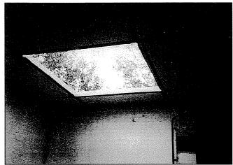
Fig. 8 Strengthening around an opening in a reinforced concrete slab at ZOLTEK Rt. in Nyergesújfalu, Hungary. (Date: Aug. 1998. Strengthening strips: Sika CarboDur M1214-25 m. Designer: Dr. Rita Kiss and Ákos Sapkás. Exec: Fischer-bau Ltd.)
