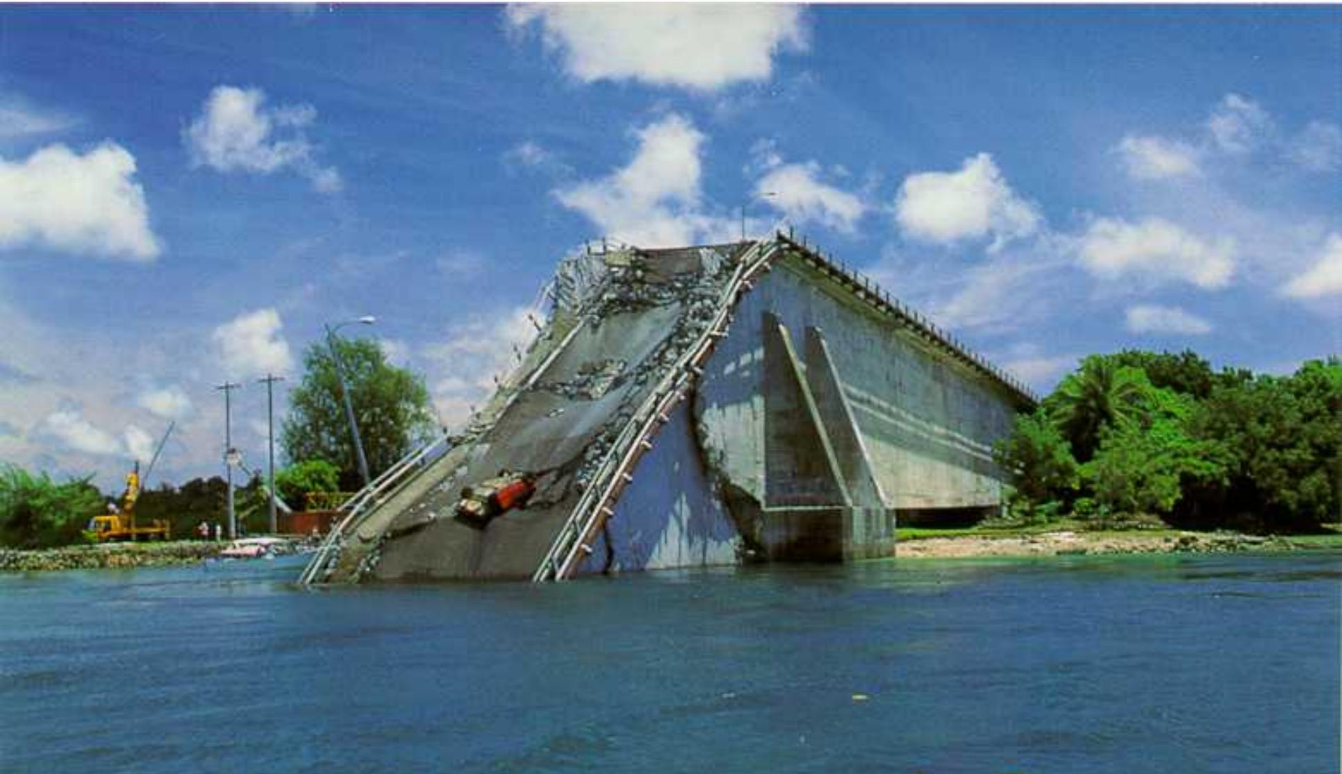
Our Verdict: Compression and shear failure, with wave from prestress failure, after creep & vertical prestress loss. Size effect must have been strong.
